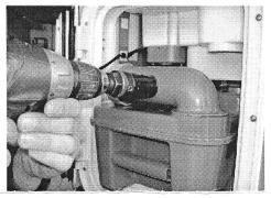
Leave cassette in service compartment and use hole miller to drill 53 mm diameter hole in outlet pipe at point marked.
